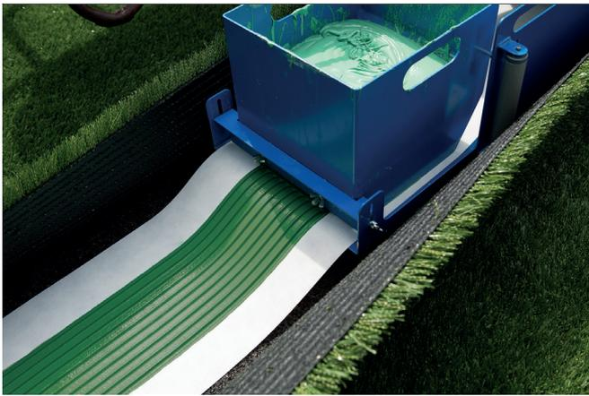
*Opening the turf, laying the seaming tape without creases, applying the adhesive and laying the turf in the bed of adhesive: the STAUF adhesive applicator machine performs all of these steps in a single process.*
