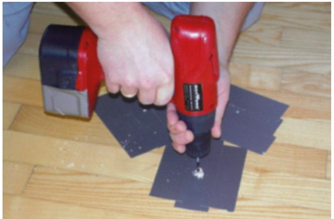
This can also prevent adhesive from escaping from the drill hole on the parquet surface. A (wood) drill diameter of approximately 2.5 to 4 mm is sufficient for drilling and injecting the liquid adhesive used here.
